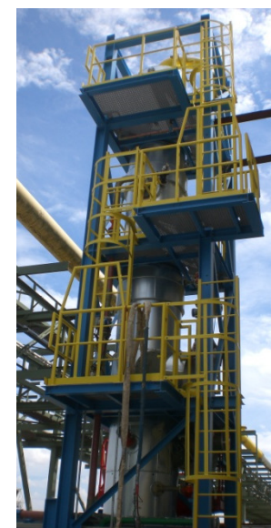
135 TDP Skid mounted \text{Cl}_2 Drying Tower
