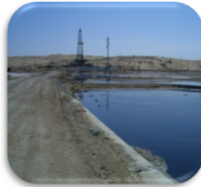
Oil lagoon sludge and sediments
